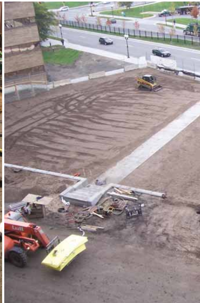
| Top grading is completed and prepared for laying sod.
