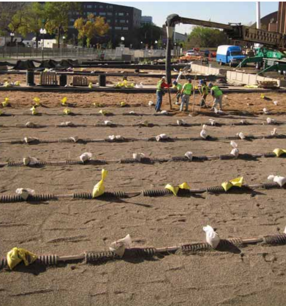
| Clean aggregate backfill is applied.
